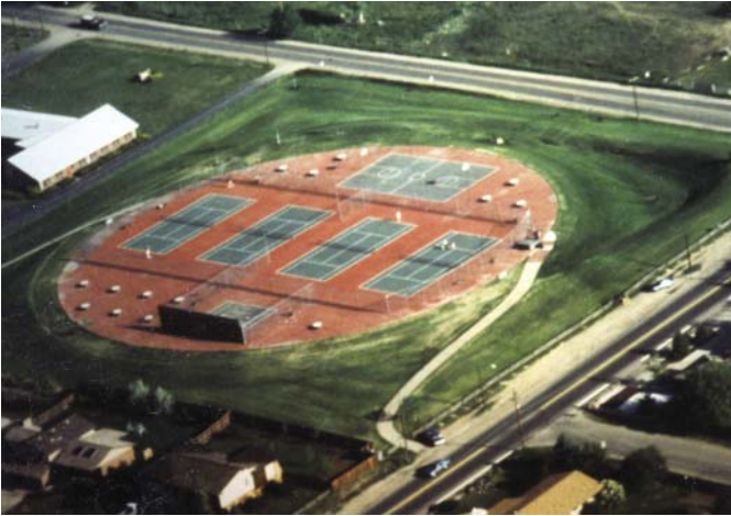
Fig. 1: Ten million gallon (40,000 m 3 ) potable water tank in Arvada, CO. Its post-tensioned roof doubles as tennis courts for visitors to the Alice Sweet Thomas Park
