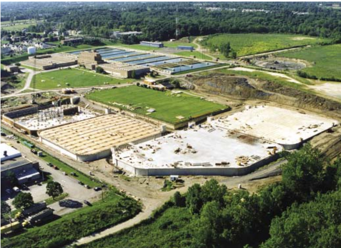
Fig. 2: The Hap Creamean Water Treatment Plant in Columbus, OH uses six post-tensioned concrete clearwells totaling over 48 million gal. (200,000 m 3 )
